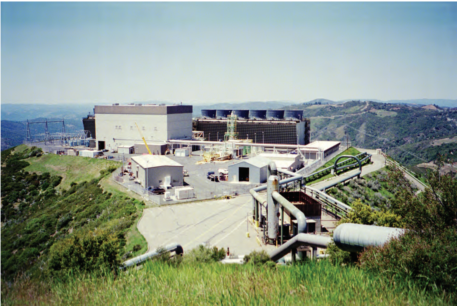
A hilltop power plant gathering geothermal fluids from the surrounding well field at the Geysers geothermal plant. The Geysers is the single-largest geothermal operation in the world with a capacity of 700MW, located about 100 miles north of San Francisco.
