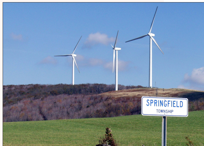
The Mill Run wind farm in Springfield Township.
